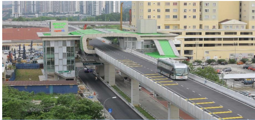
Electric Buses for BRT
